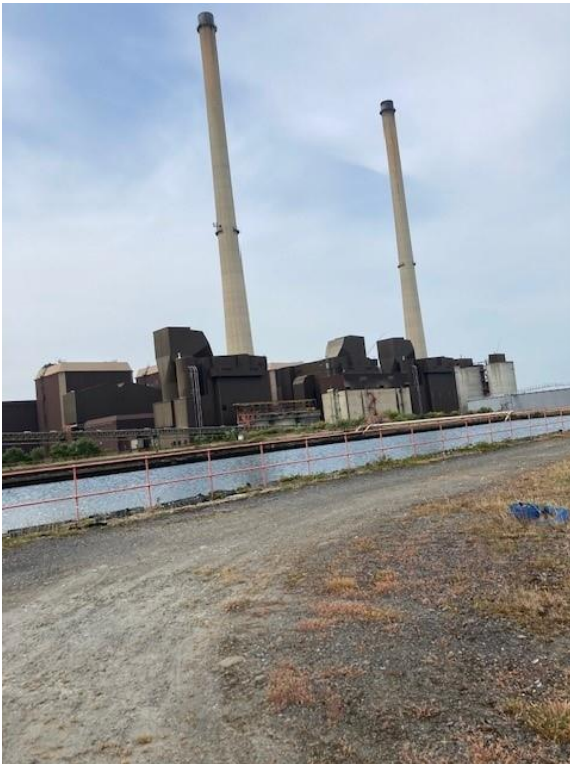
Photo 3.9: Service Reservoir in located within the Moneypoint Generating Station
