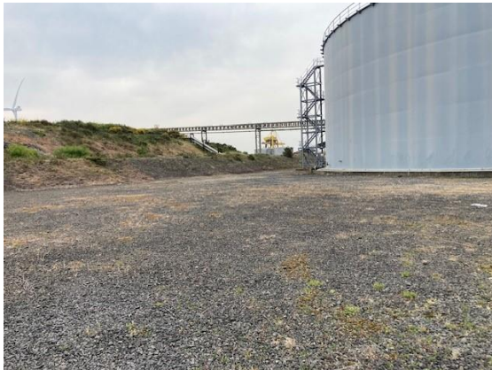
Photo 3.2: Building and surrounding gravelled surface within the Moneypoint Generating Station
